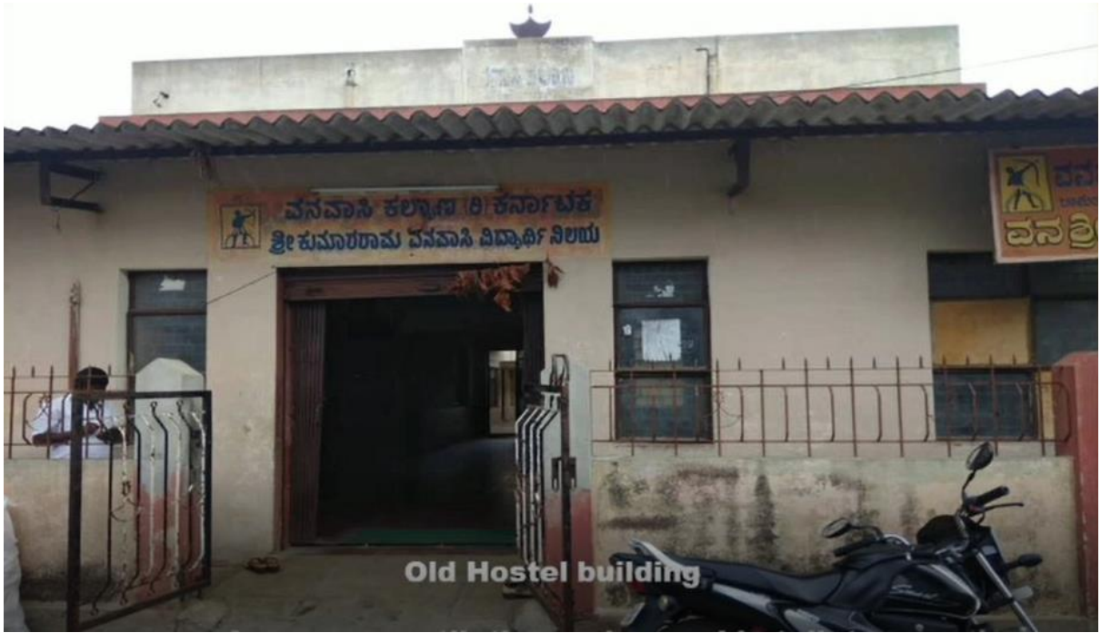
Old Building (Before demolition)
